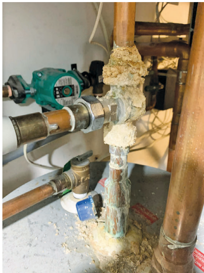
A system with reduce fluid conductivity will minimize galvanic corrosion, which has taken over the fitting/pipe.
