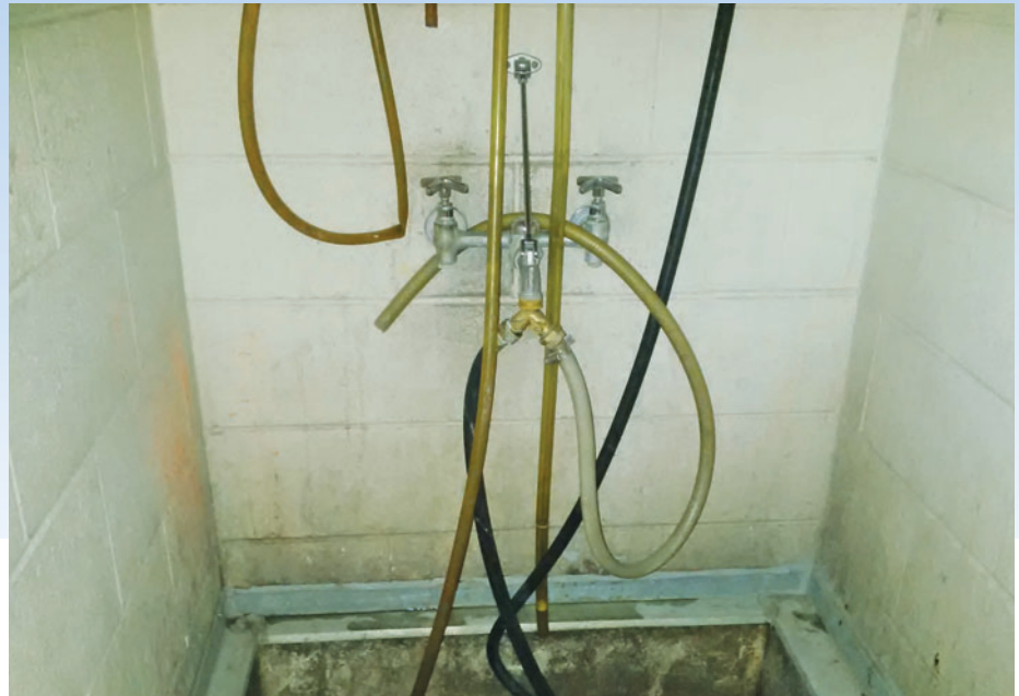
Metal particulates in the system can cause corrosion as seen in this sink.
